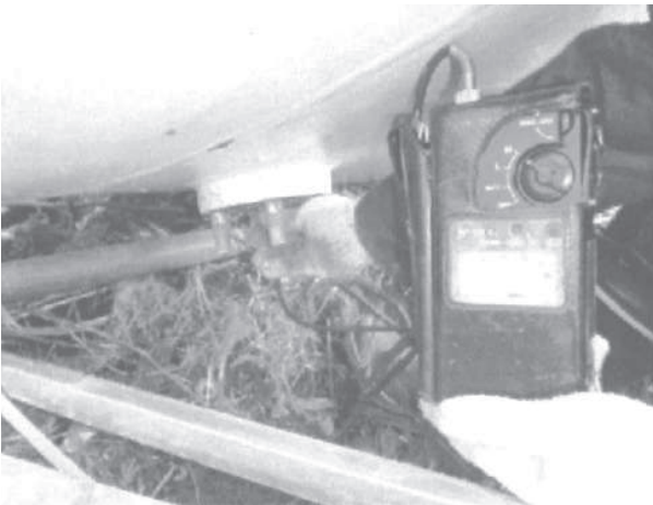
図3-7 LPGガス濃度0%を確認
